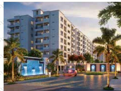
Avinash Metropolis Khoka-Junwani Road, bhilai
